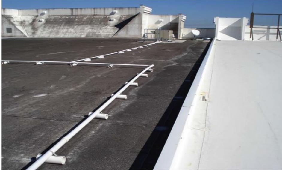
The roof can shrink, too, making it more vulnerable to hail damage and difficult to heat weld during repairs.
